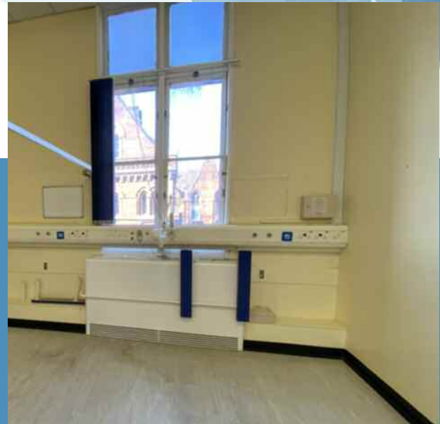
Ward 37: Pictured before the refurbishment to accommodate COVID-19 patients.
